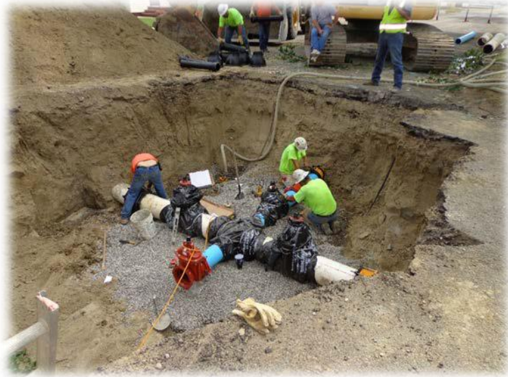
Installing New Waterlines in Roundup
