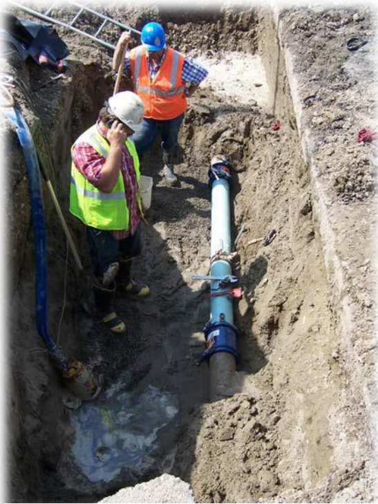
Water Line Repair in Roundup
